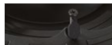
Stainless steel fixing screws with Neoprene covers
