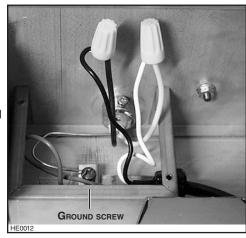
IN-LINE OR EXTERIOR BLOWER: Remove rough-in plate wiring cover and connect wiring (see instructions included with in-line or exterior blower).
