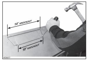
Removing vertical knockout opening on rough-in plate.
