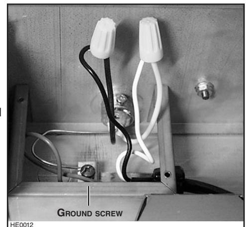
IN-LINE OR EXTERIOR BLOWER: Remove rough-in plate wiring cover and connect wiring (see instructions included with in-line or exterior blower).
