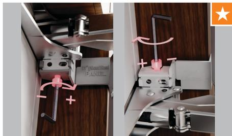
Open the door and use the supplied hex key to expand the spacers. Ensure no gaps are present.
