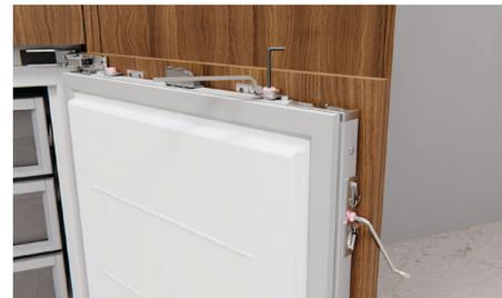
Fit side screws to panel using the short crosshead tool provided in the install kit. For 90° door opening installs, the supplied crosshead key should be used on the hinge-side.
