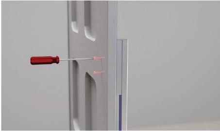
Determine the panel orientation based on the hinge and handle positions. Red labels indicate left hinge installations, blue labels indicate right hinge installations.
