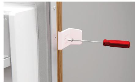
Unscrew the crosshead screws to remove depth gauges. Set aside.
