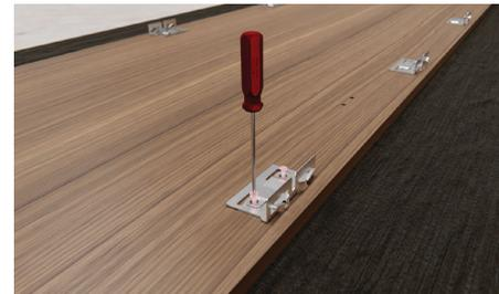
Secure the side brackets using two screws per bracket. Ensure side brackets are fitted tightly and the fasteners are secured straight.
